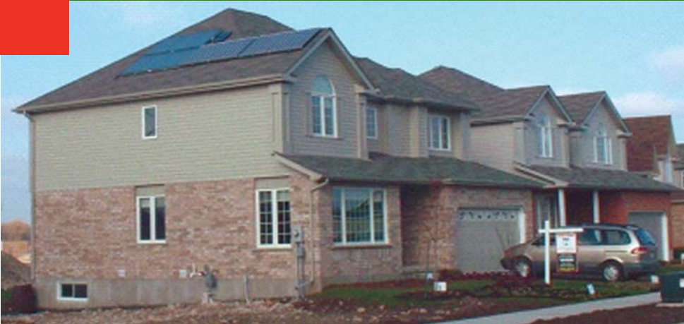
Figure 1 – The Southfield home in Guelph, Ontario modeled passive solar design for free heating, cooling and lighting; an active solar domestic water heating system; a grid-tied photovoltaic (solar electric) system; and energy-wise landscaping. One year of monitoring revealed the solar systems produced comparable quantities of energy as conventional energy upgrades, for comparable costs.
